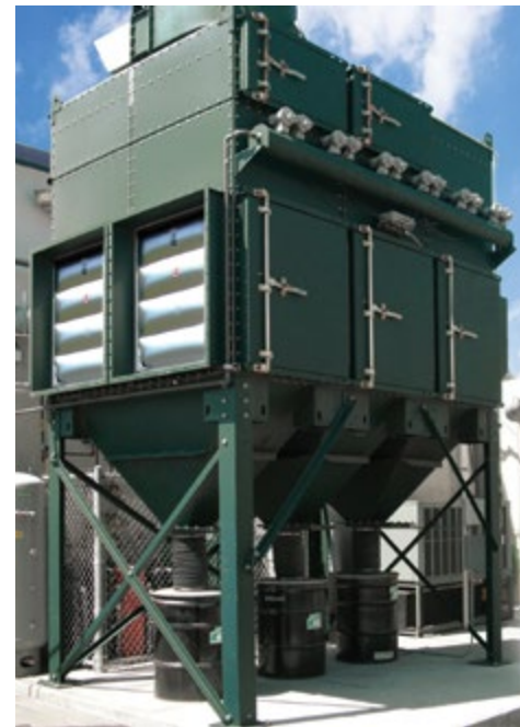
Dust collection systems should include protection equipment, such as explosion venting. A dust explosion in an unprotected dust collector produces a high-pressure wave that can fragment the housing and send heat, flames and dangerous projectiles into the surrounding area. (Image courtesy Camfil APC)
