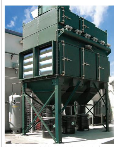
Dust collection systems should include protection equipment, such as explosion venting. A dust explosion in an unprotected dust collector produces a high-pressure wave that can fragment the housing and send heat, flames and dangerous projectiles into the surrounding area. (Image courtesy Camfil APC)
